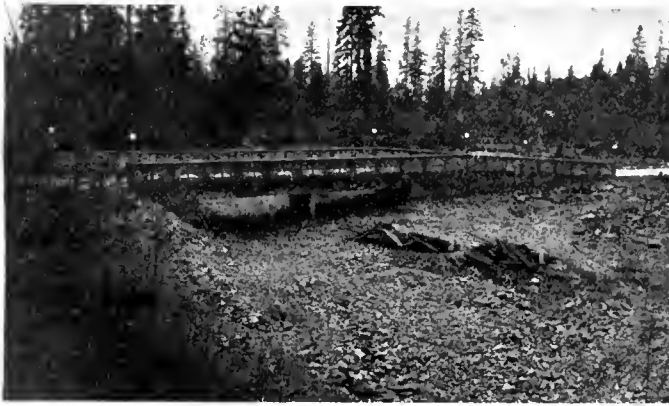
Reinforced Concrete Bridge, Marine Highway, B. C.
